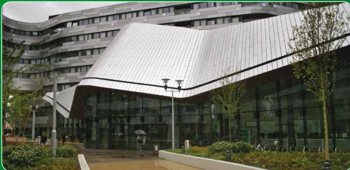
Vanbrugh Community Pain Management Clinic, Greenwich
